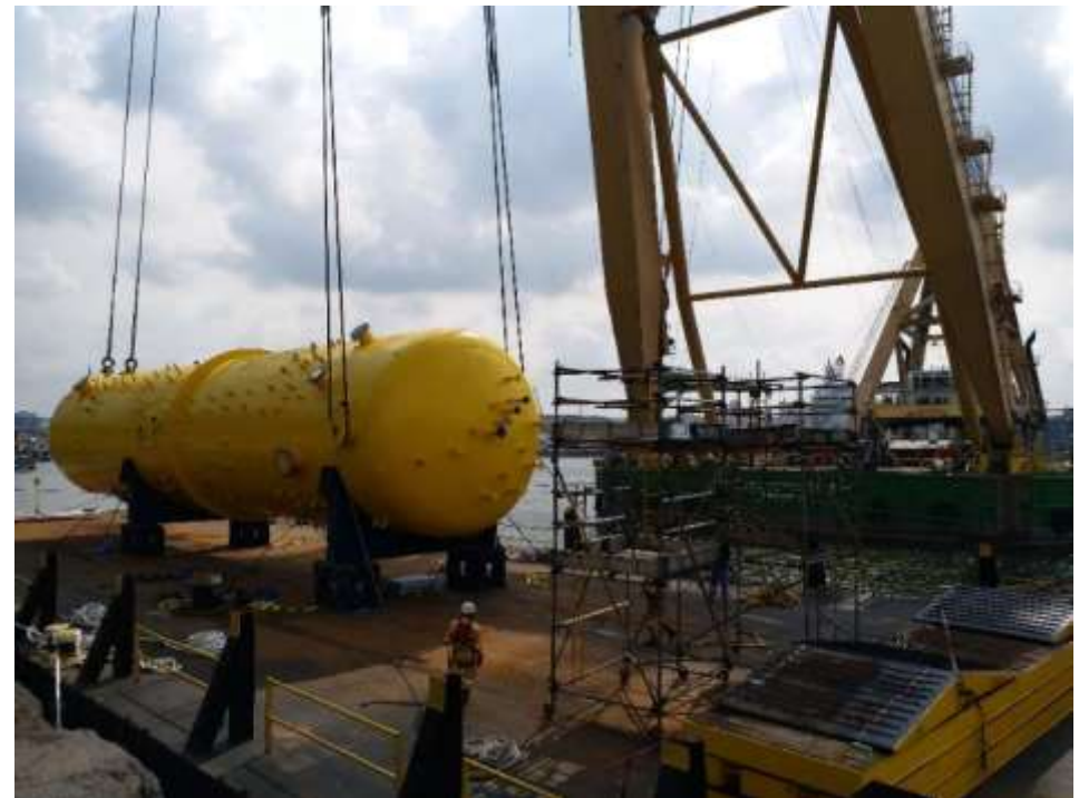
Loading of Water Treatment Skid At Jurong Port
